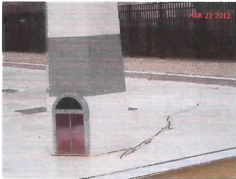
Cracks evident are deep and numerous photo dated March 22, 2012
