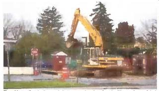
The old gasoline tanks are being removed and replaced with county-mandated double-walled tanks at Isilp Town's East Isilp Department of Public Works yard to 100 Cartton Avenue.
